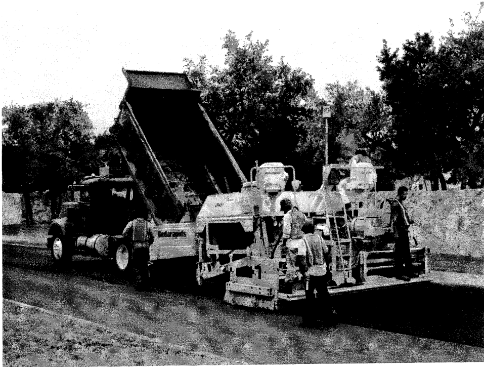
Figure 8-5 Asphalt paving machine in operation. (Courtesy of Cedarapids, Inc.)
