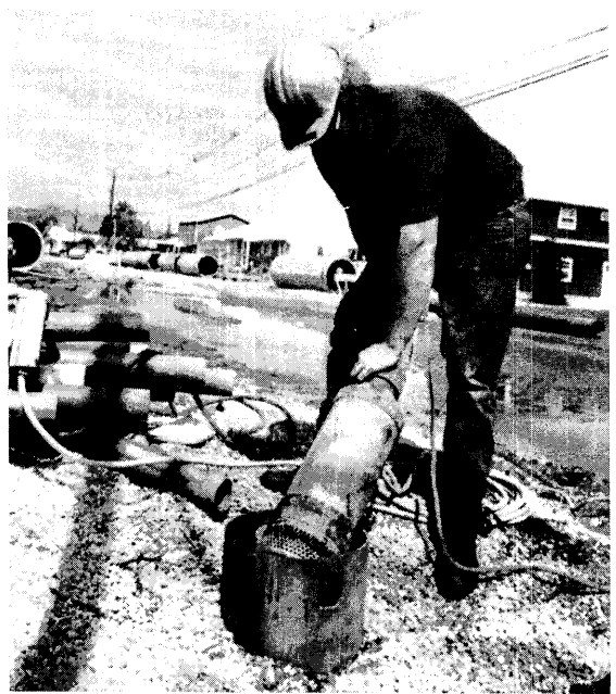
Figure 10-23 Electrically powered submersible pump being placed into dewatering well. (Courtesy of Crane Pumps and Systems)
