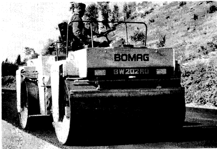
Figure 8-8 Rolling an asphalt pavement with vibratory roller. (Courtesy of BOMAG [USA])
