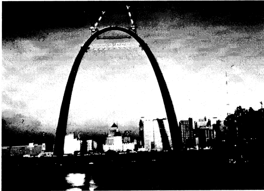
Figure 1-1 Construction of St. Louis Gateway Arch. (Courtesy of American Institute of Steel Construction)
