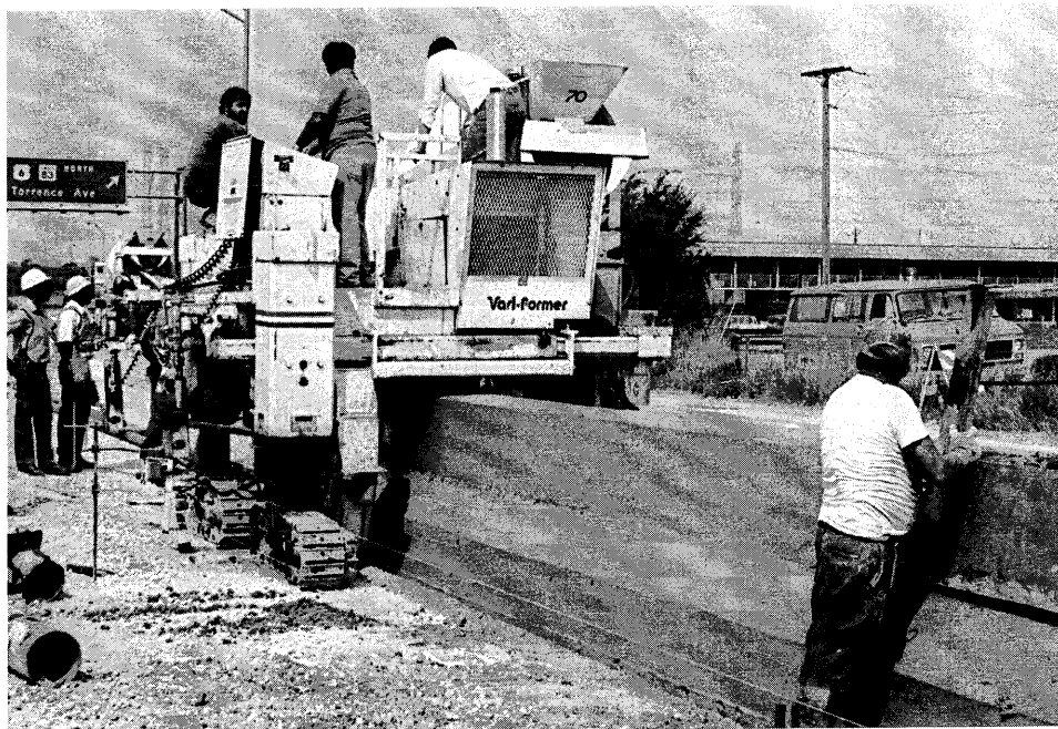
Figure 8-3 Slipform paver placing median barrier. (Reprinted Courtesy of Caterpillar Inc.)
